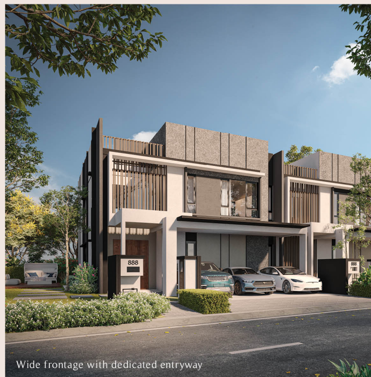
Unique façade with lasting symmetrical architecture
